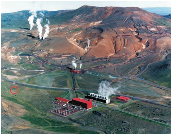
Figure 2. A view to the Krafla Central Volcano. A 60 MW power plant is seen in the foreground. The red circle denotes the potential IDDP drill site (Photo by Emil Thor, Iceland).
