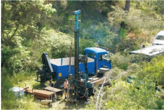
Figure 2. Drilling operations at section LB1 with a trailer-mounted rig.
