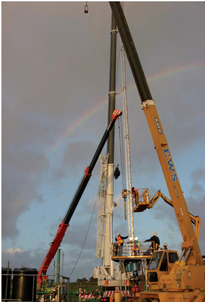
Figure 5. Multi-crane lift deployment of 32 m-long bottomhole assembly consisting of U-tubes, seismic sensors, and pressure temperature sensors at the CO2CRC Otway Project Site, Victoria, Australia.
