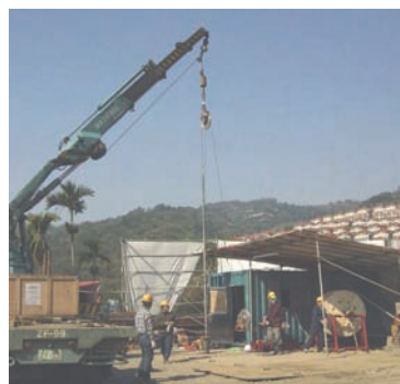
Figure 1. The precise temperature instrument that was installed in the well head of TCDP Hole A.
